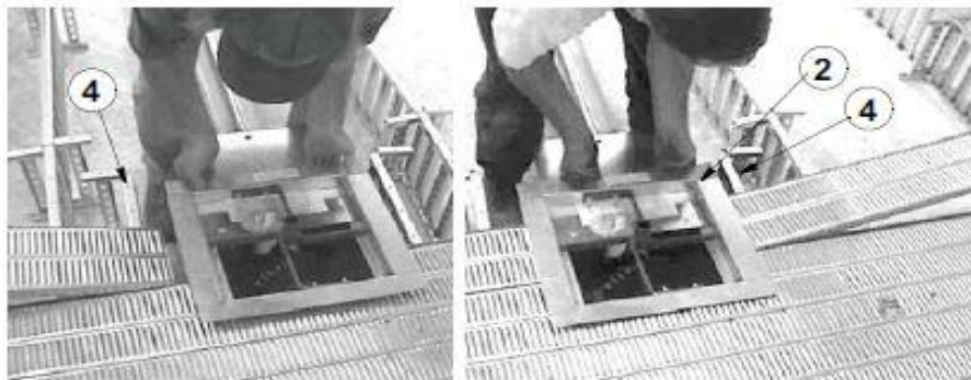
Figure 27. Floor Planks at the Sump
