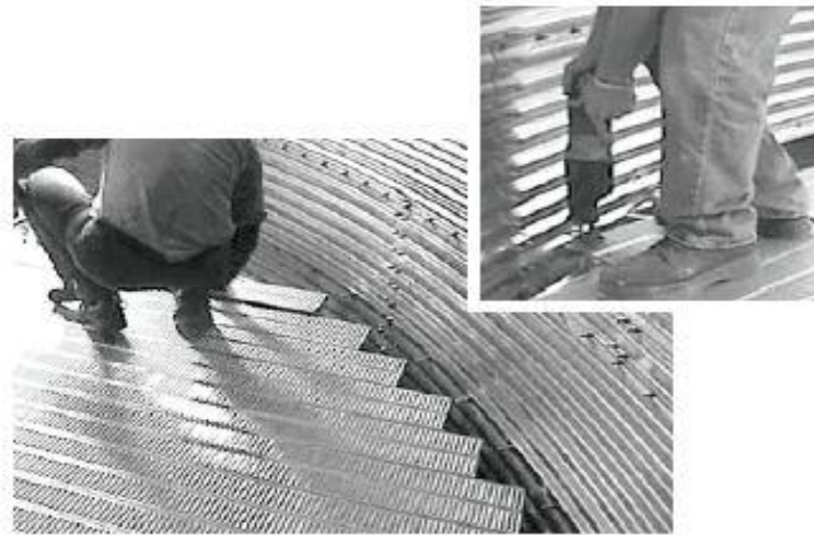
Figure 31. Final Plank Length Adjustment
