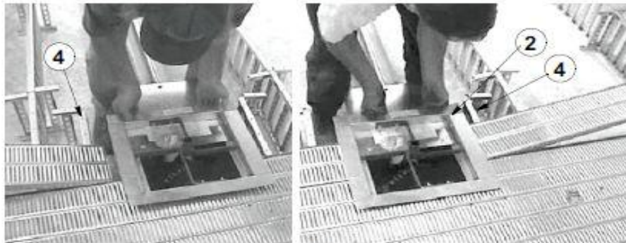
Figure 27. Floor Planks at the Sump
